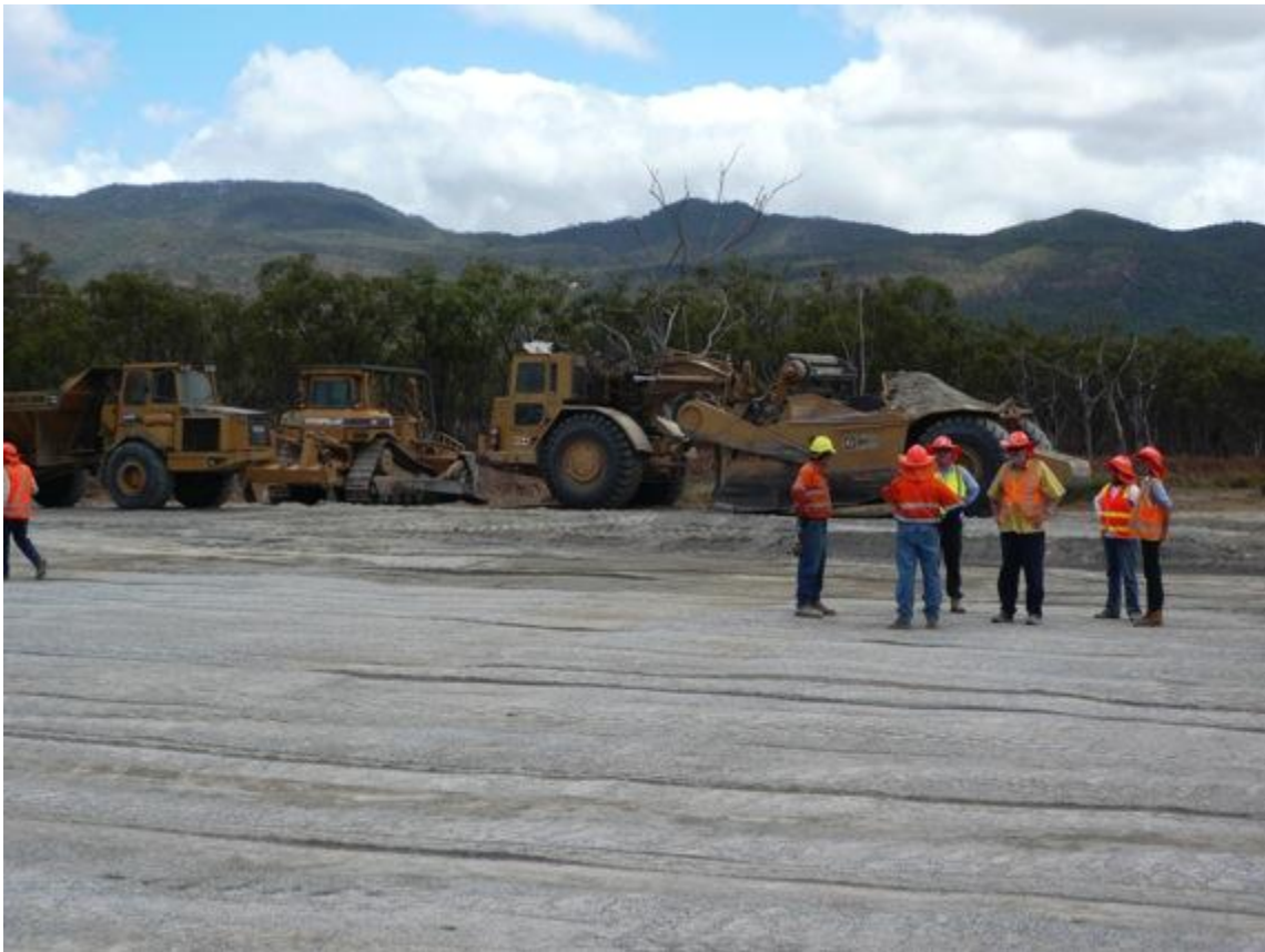
Carbine Tungsten Board of Directors Inspecting the Tailings Retreatment Construction Site
