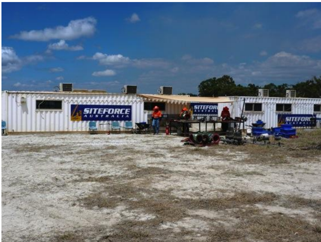
Construction Team Reconditioning Pumps, Valves and Kelsey Jig Plant
