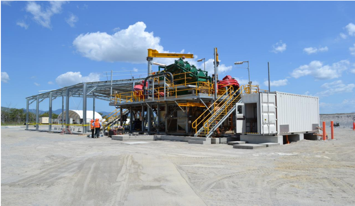
Figure 1. Mt Carbine Tailings re-treatment plant between the Mulligan Highway and No 4 Tailings dam on 12 January 2012, showing container/MCC at the right, Kelsey Jig modules in the centre and shaker table shed nearing completion at the left of plant complex.
